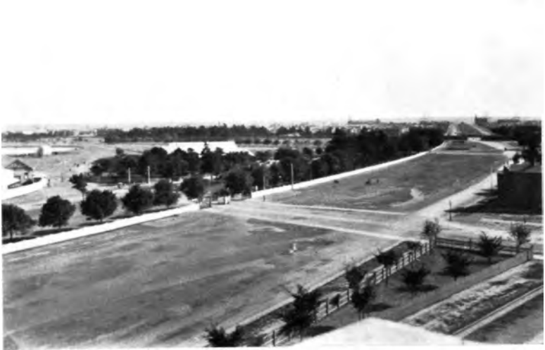
View of Albert Road looking West, 1900.
