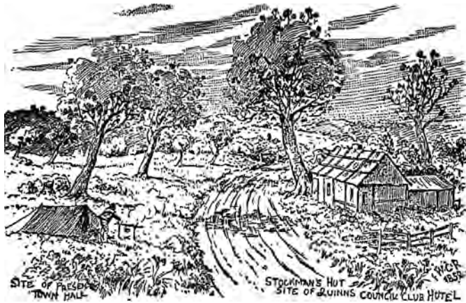
Road from Liardet's Beach to Yarra River, 1852.
