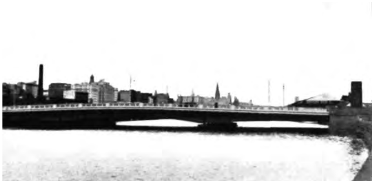
Spencer Street Bridge.
