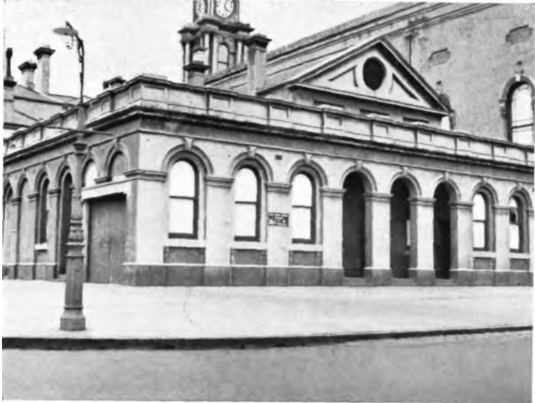
Police Station and Courthouse, 1880-1928, Town Hall Buildings. Now Baby Health Centre, South Melbourne.
