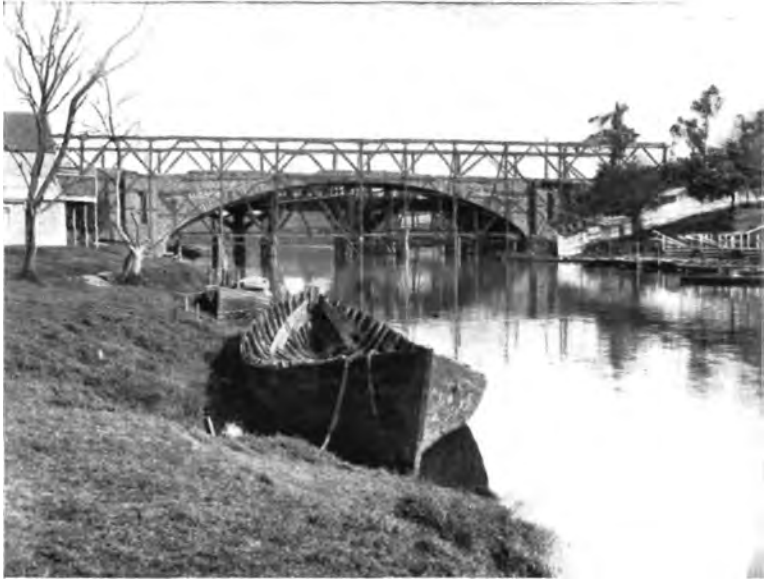
First Prince's Bridge before completion.
