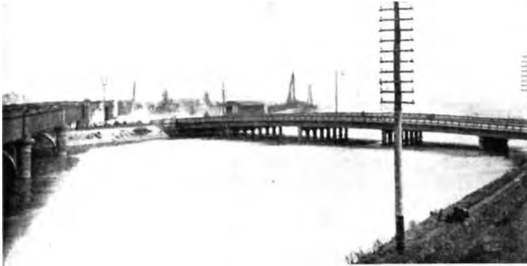
Railway Bridge (left) and Queen's Bridge over the Yarra River.
