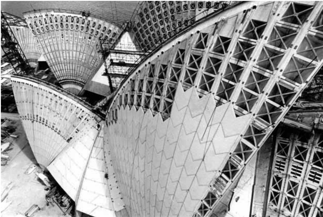
Figure 11. The sails during construction.
