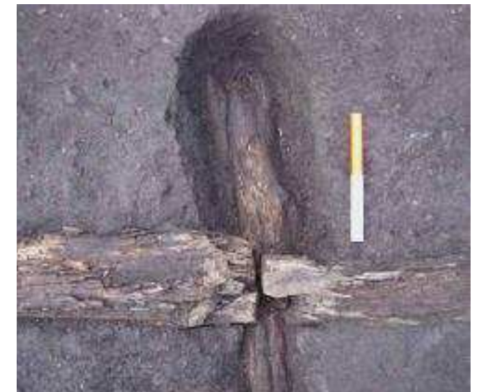
16. Detail showing two rails pegged into an irregular sleeper on the Harraton Colliery Waggonway (PCA 2010: Plate 11 - Area A, Rails 217 and 218 on sleeper 193 in waggonway 180). Photograph courtesy of Pre-Construct Archaeology
