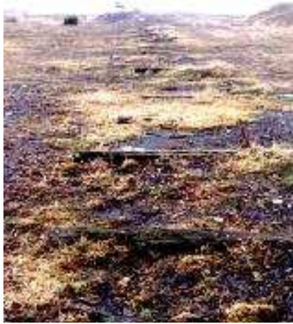
13. Wooden sleepers of the latest phase of colliery railway at Weetslade, North Tyneside. Carlton 1998
