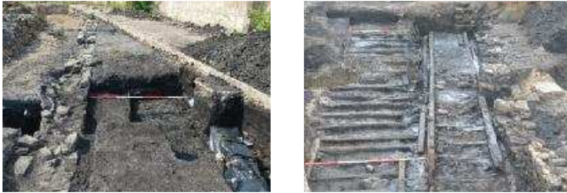
35. The Carville Hall boundary wall ( left ) running to the northern boundary of the site.
