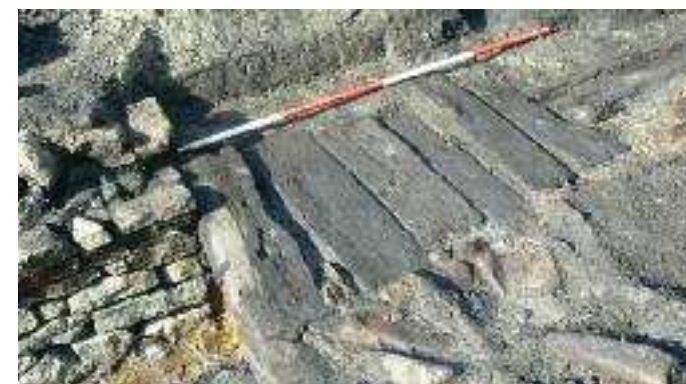
61 Transverse planking capping the south end of the leet.
