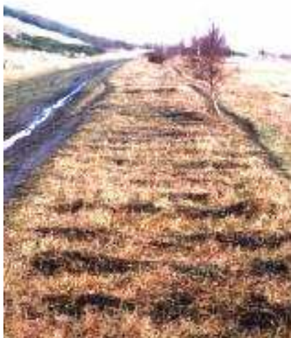
14. Undulations in a former trackbed where sleepers have been removed from a former colliery railway at Weetslade. Carlton 1998
