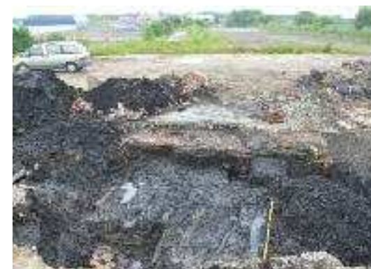
26. Sleepers uncovered on the east side of the Carville Hall boundary wall with the remains of a brick floor, part of the Tyne brickworks, on its west side.
