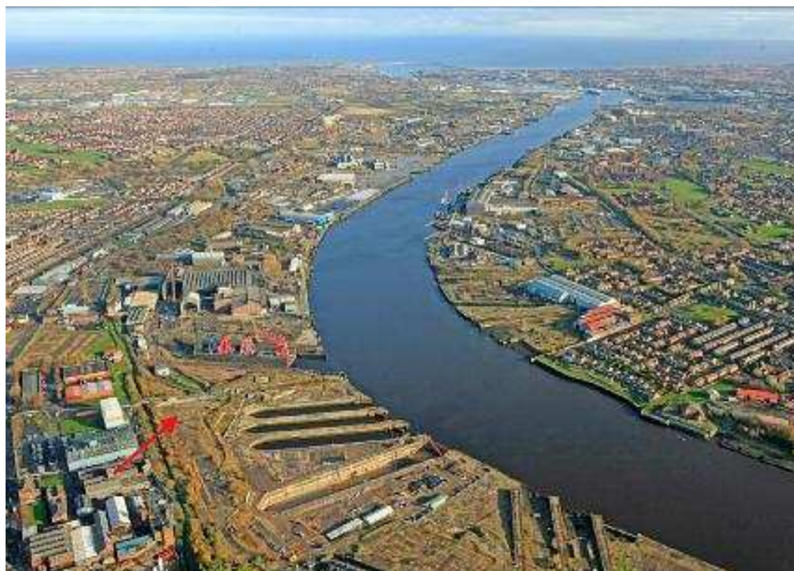
2. Aerial view of the Neptune Yard site in 2013, viewed from the west, showing the excavation site (arrowed), cleared of buildings prior to excavation and with the Ship Inn, site of the Segedunum Roman bathhouse, still standing 100 metres east of the waggonway site.
