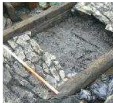
47 Part of the horse-way cobbled surface lifted to reveal well-preserved sleepers beneath.
