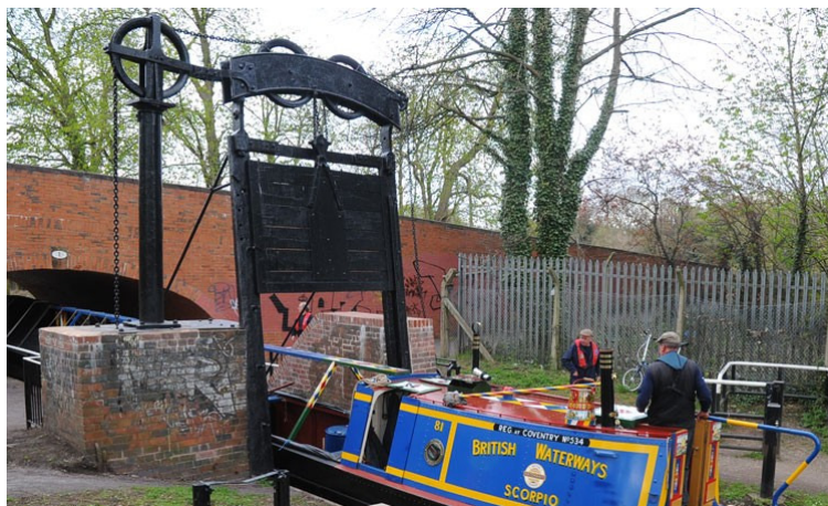
An example of a vertical lock gate
